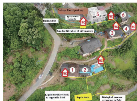
▲ The Rural Environmental Management Science and Technology Innovation Alliance demonstrated the reconstruction and improvement of toilets in highly populated areas in Dalao Village, Guizhou Province
